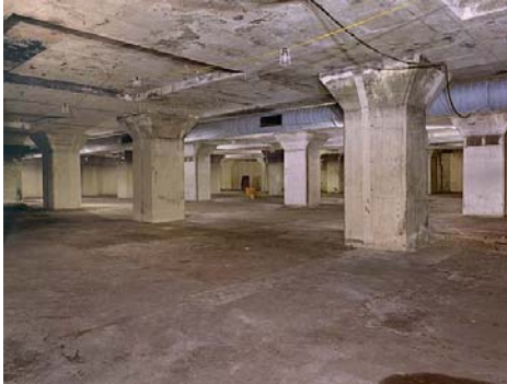
Photo: The upper floor (basement) at Station Z. The ventilation trunking suspended from the ceiling is a recent addition. Photo by Nick Catford
