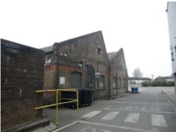
The 1898 factory building
