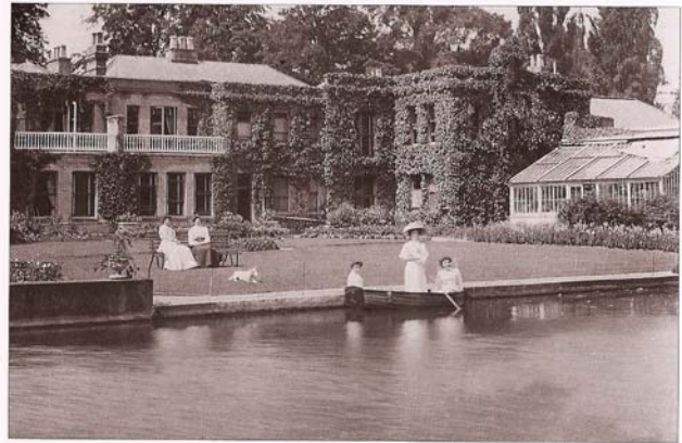
73 This romantic scene is of the house servants enjoying the facilities while the owner, John Hogg, was away. Most of West House was 19th-century in date. The whole of the creeper-clad section, and the part with the right-hand balcony, has gone.
